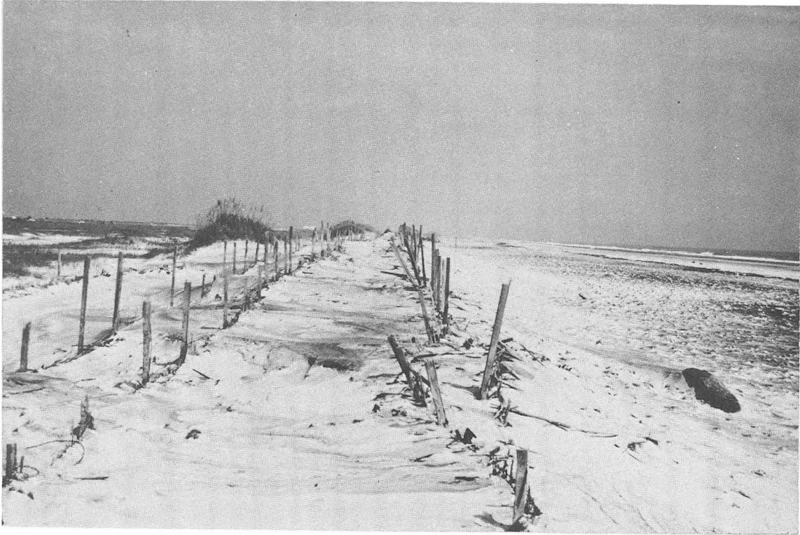
Figure 6-32. Sand fence deterioration due to exposure and storms.
