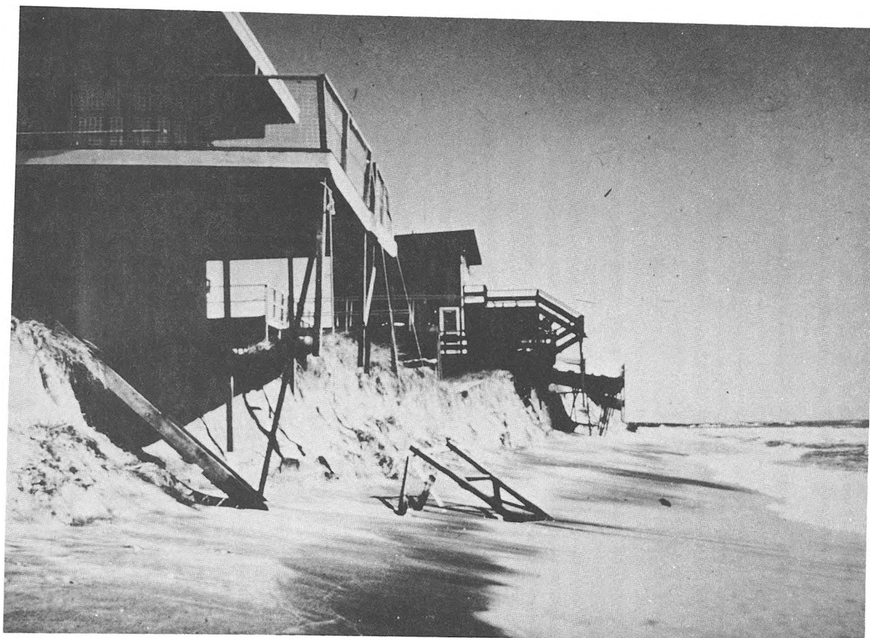
Figure 1-11. Undermining of structures by storm waves, Potham Beach, Maine.
